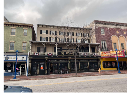
EXISTING FAÇADE PHOTO
