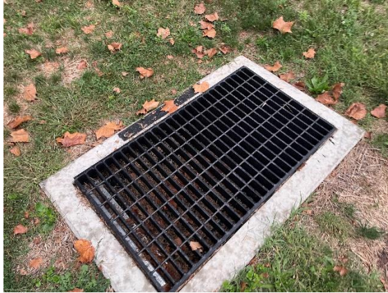
Stormwater drain on TMP 15-4-8.3
