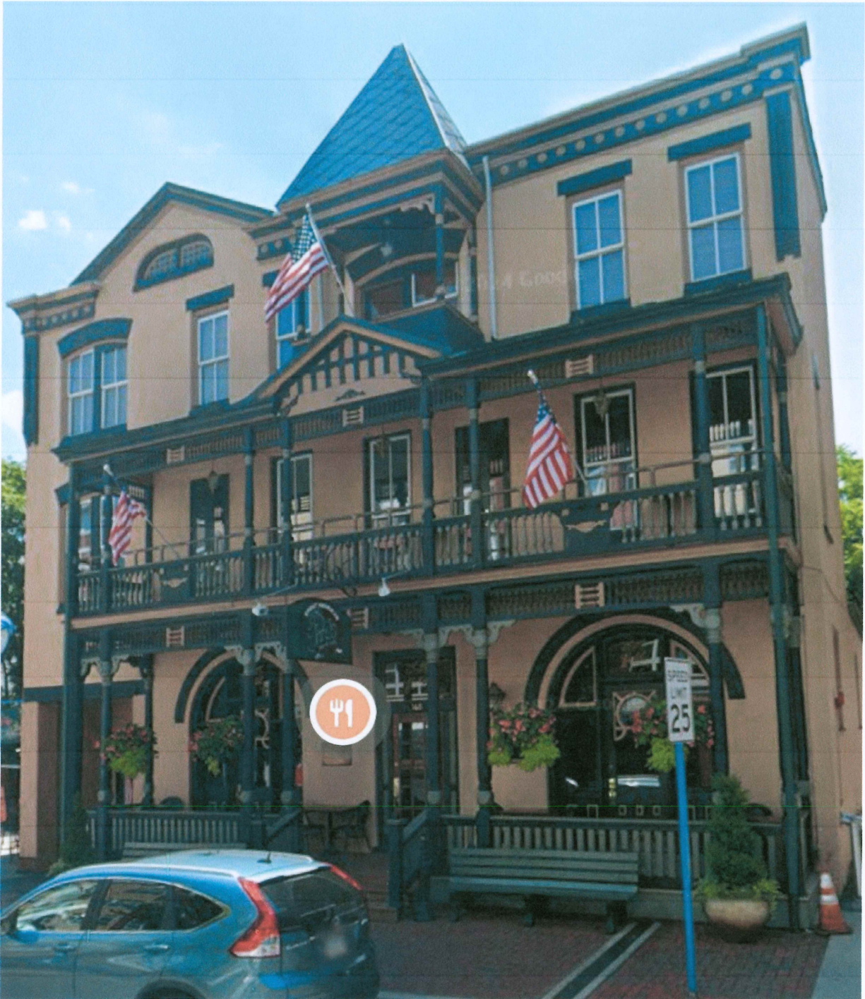
Photograph 6: Existing Historical Decorative and Structural Wood Carpentry Before Repair Work
