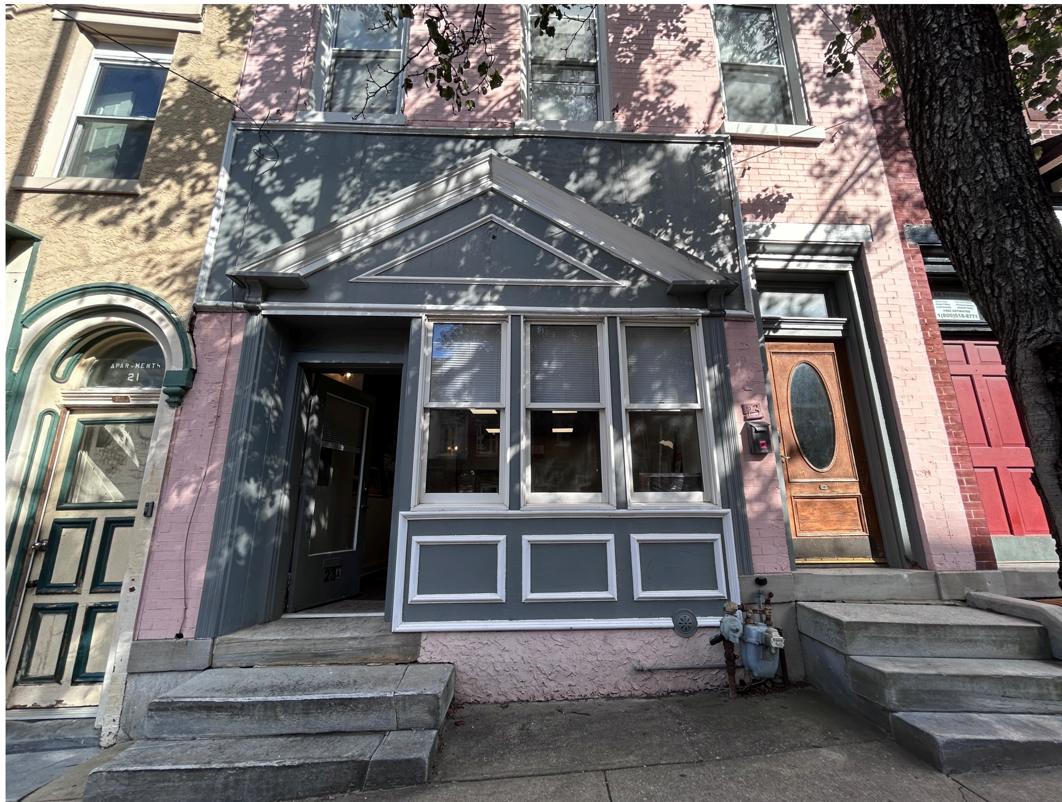
EXISTING MAIN STREET PHOTO
