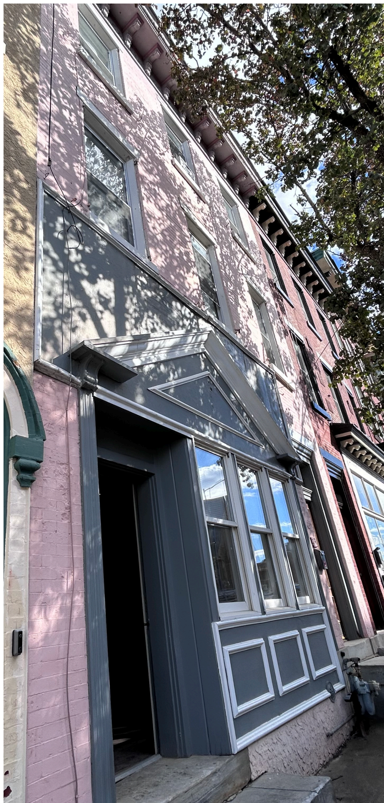
EXISTING MAIN STREET PHOTO
