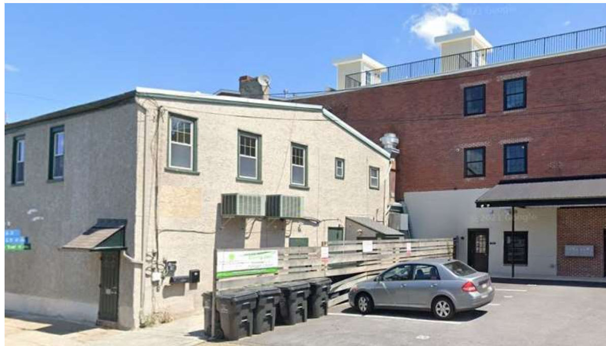
BACK CORNER VIEW BEFORE CONSTRUCTION
