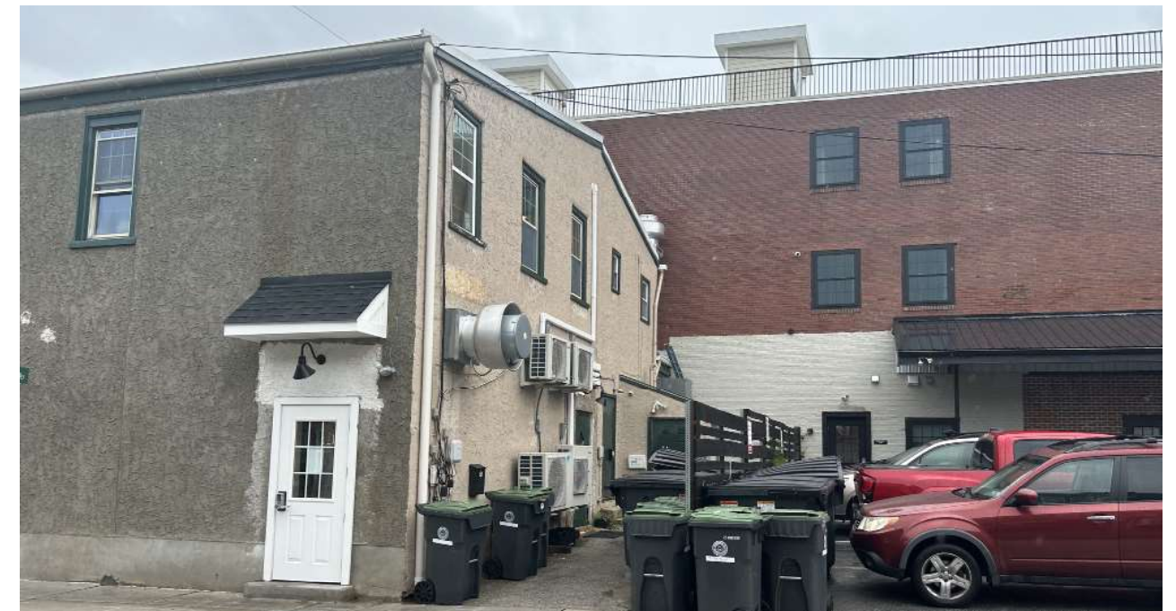
BACK CORNER VIEW AS OF AUGUST, 2024
