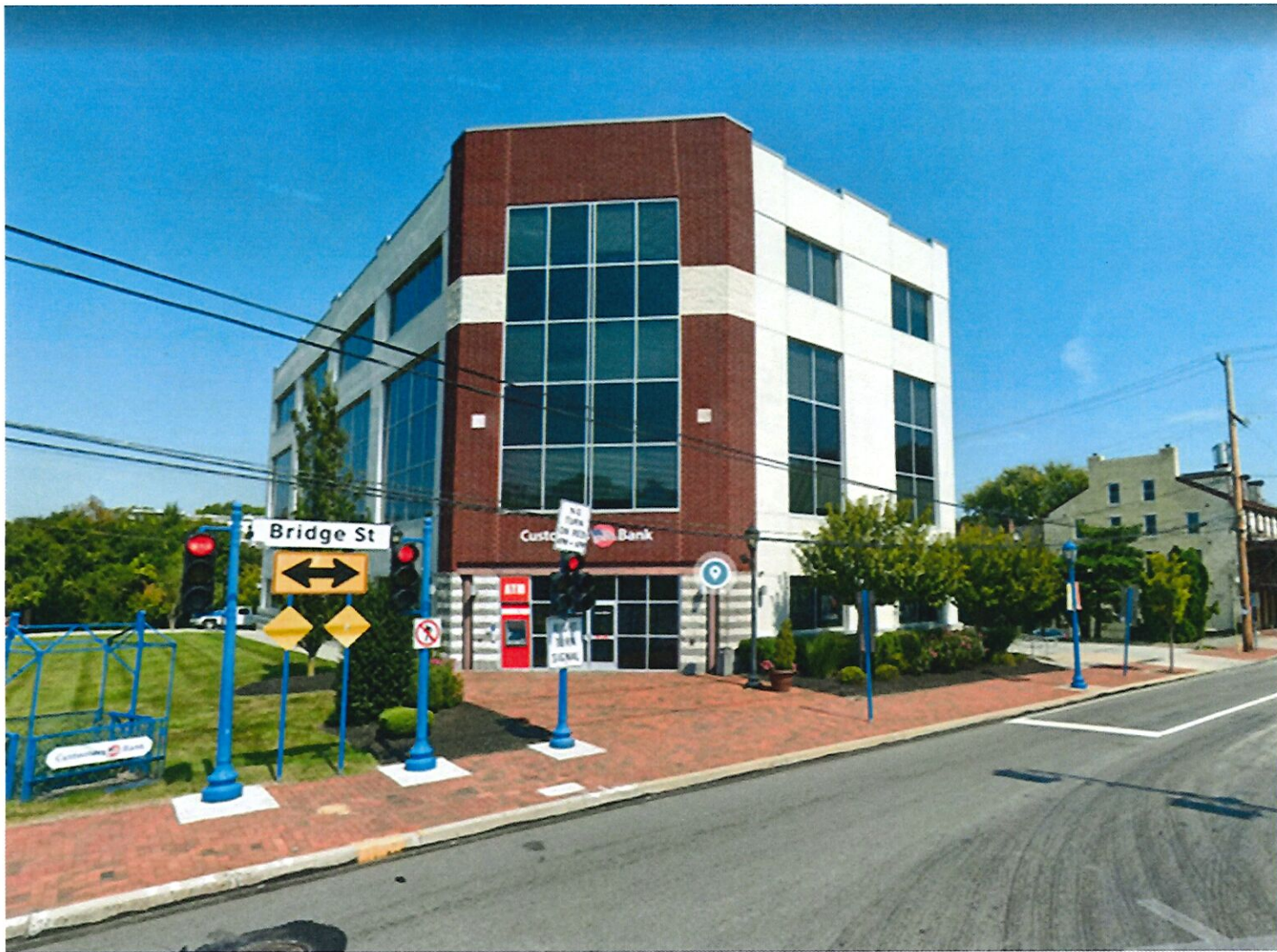
Bank across from Bluebird – Bridge & Starr Streets
